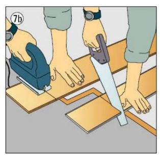
**STEP 7** Measure and cut-off the last panels of the first row. The cut-off materials from the first row can be used to begin the second row, but it must be more than 12" (300mm) in length.
